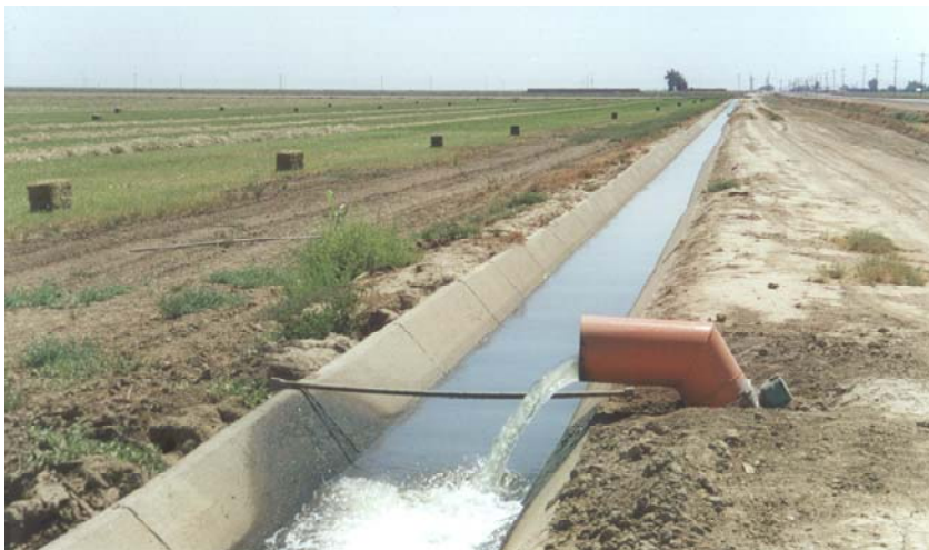
Panoche Water District: Discharge of agricultural drainage from a tile drain to an irrigation canal. Photo: Susan Austin
