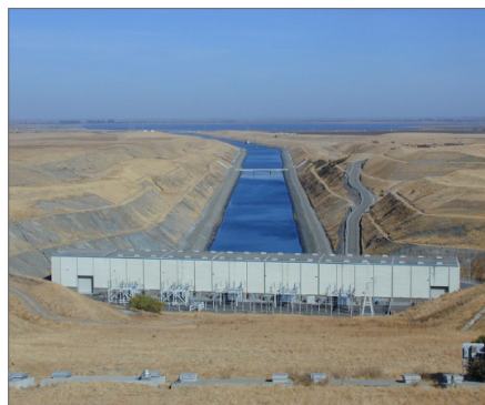
Massive pumping plants in the south Delta draw in water for export. | Both photos Courtesy of Diana Jacobs, SRPT
